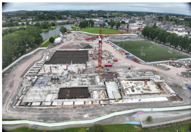
Overview of site
