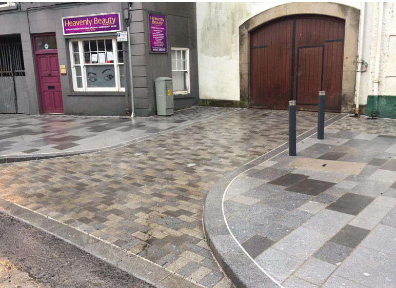
East Bridge Street- Courthouse vehicle entry
