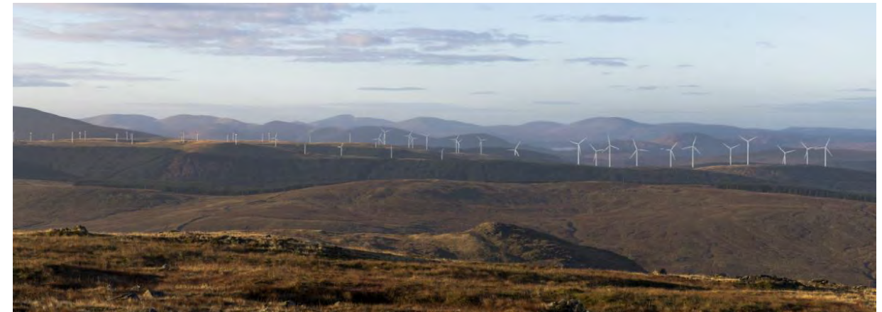
Windy Standard I and III Windfarms, Dumfries and Galloway (Photomontage): three sizes of turbine (55m, 125m and 177.5m. Seen from Blackcraig Hill the differences in size are clear
