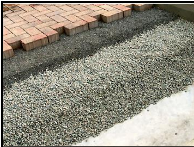
Figures 2-3 - Cross section and example of typical permeable pavement
