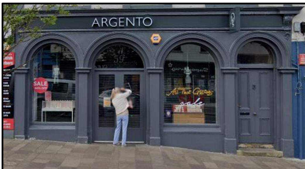
Figure 4: Acceptable shutters showing internal grille. (Market Street, Omagh)
